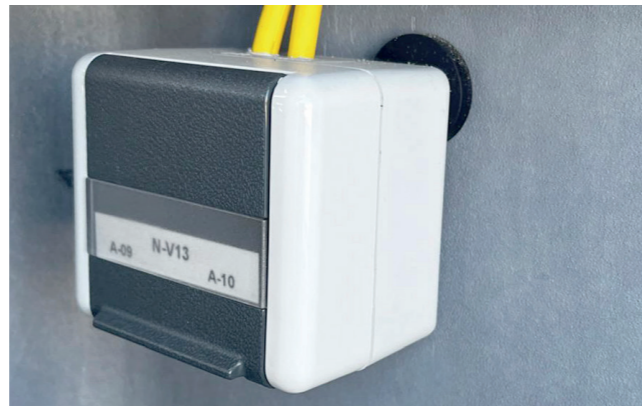
Install sockets directly on the steel girder
