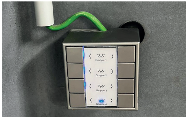
Mounting switches and control panels
