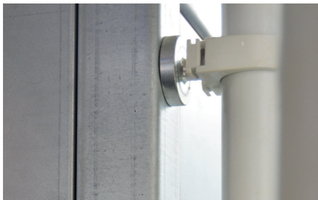
Fastening cable ducts magnetically
