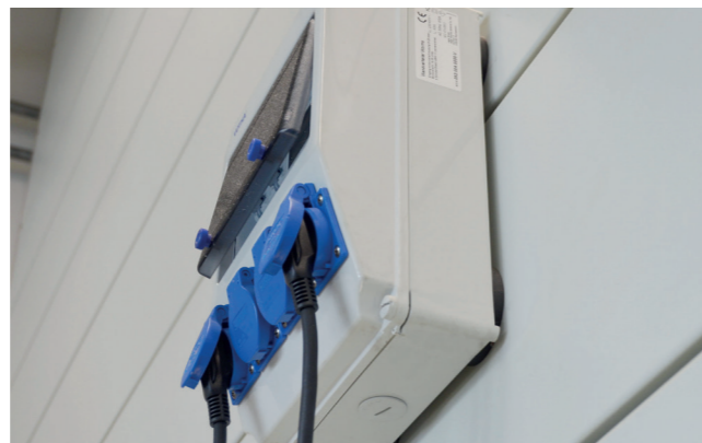
Fastening switch cabinets or sockets magnetically
