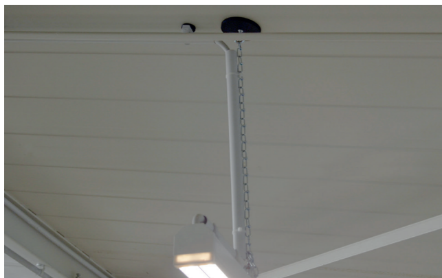
Suspending lights from the ceiling
